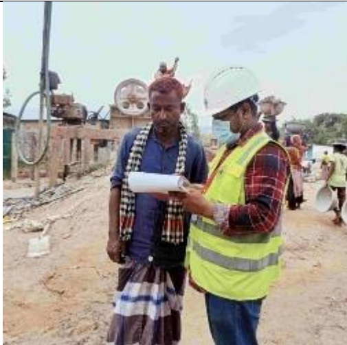
Consultation with Crushing Operator at Bholaganj land port area
